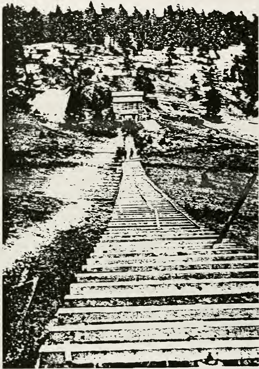
Figure 23. Revenue tramway, ca. 1899. Building in distance is not mill, but a ore holding structure located up the hill and east of the mill. (Photograph courtesy of Bill and Doris Whithorn, Park County Museum, Livingston, Montana.)
